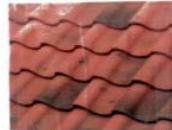
Clay pantiles on roof area of cart-lodge plot 4.
